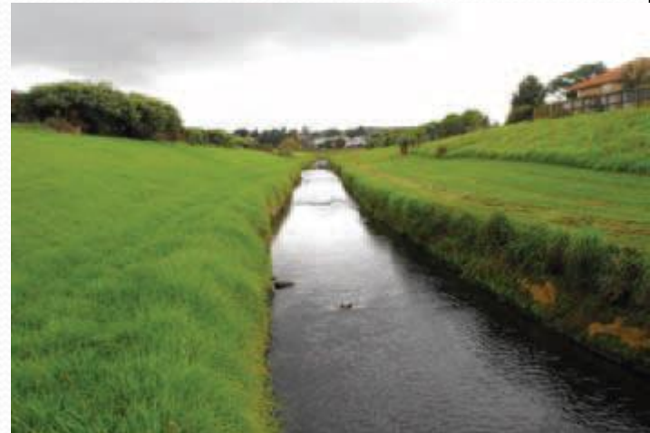
Channel straightened and deepened
