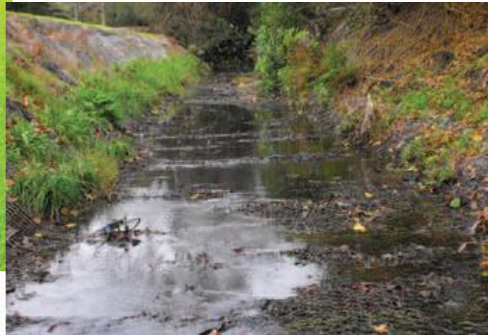
Bank and bed lined with permeable artificial lining
