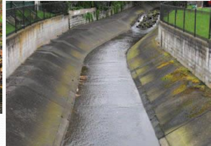
Bank and bed lined with impermeable artificial lining
