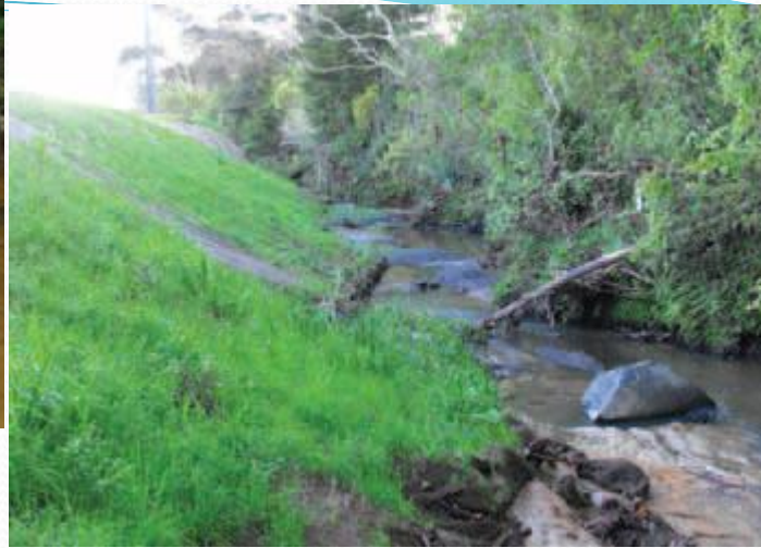
Upper bank widened to increase capacity
