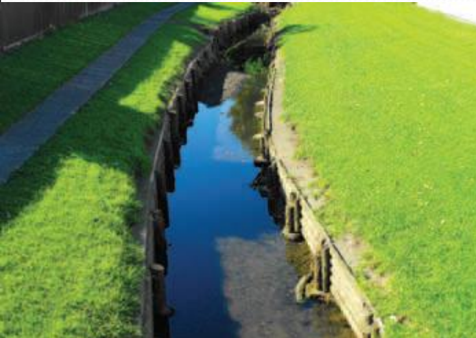
Banks lined with impermeable artificial lining
